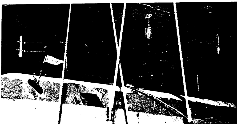
b. Internal tendon grout injection port
